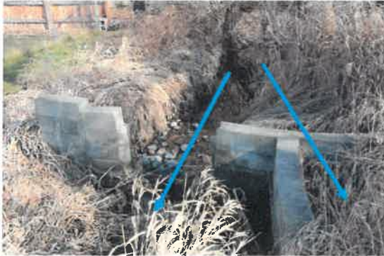
At Point #2 looking northeast
