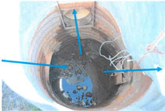
Inside view of the vertical pipe from the above picture.
